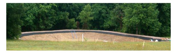
The final size of our pond is 100' long by 60' wide. Outside the pond area, the contractor found a natural spring and dug a well. We set up a submersible pump inside the well with an external on/off switch and piping to the pond.
