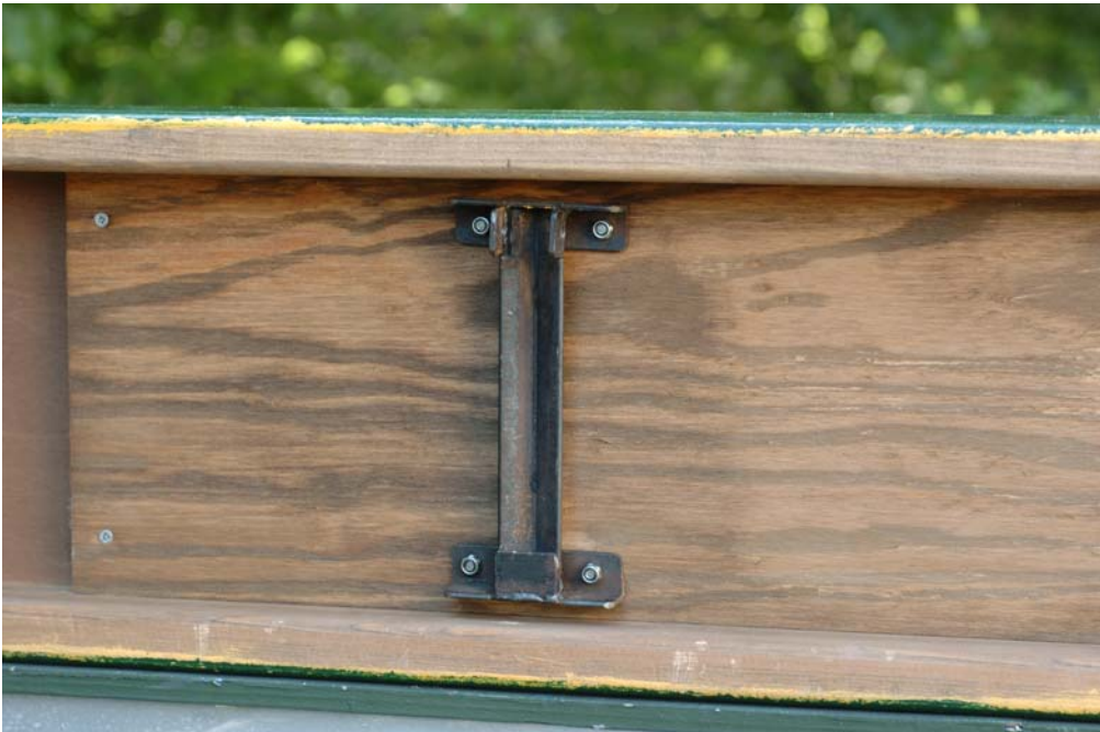
Figure 5B Angle Plate Component of Fulcrum of Premier Board
