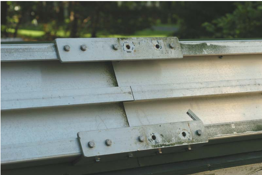
Figure 3B Max 200 M-Board Attachment Plates
